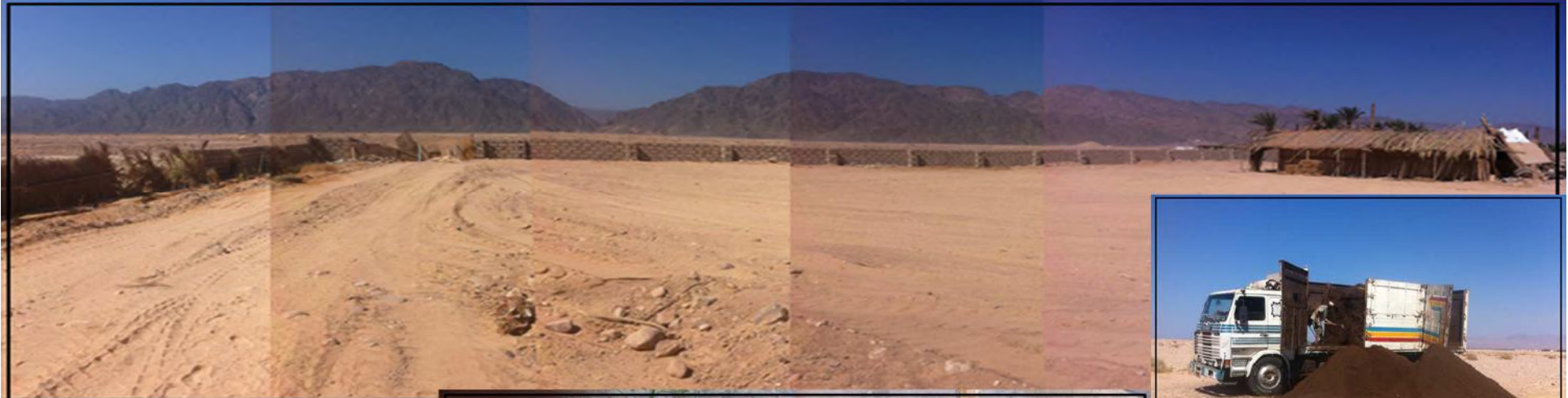
CLEARED PROJECT SITE
